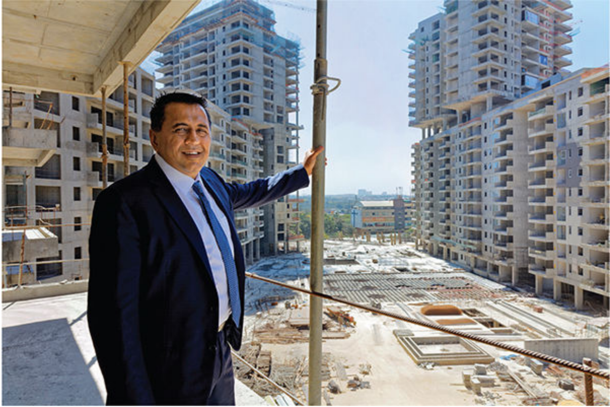
Jitu at the Embassy Lake Terraces project site
